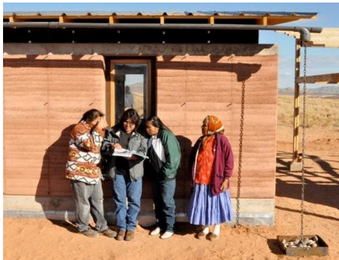
As architecture students from the University of Colorado Denver, these AmeriCorps volunteers worked with Design Build Bluff to build housing for Navajo families. Photo by Wes Hoffman
